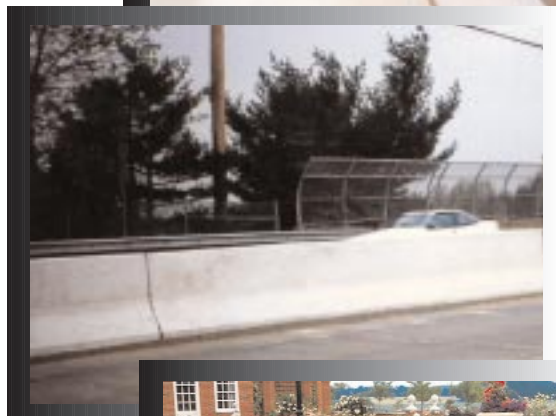
Fig. 8. White traffic barrier sections are bright and highly visible to drivers.
