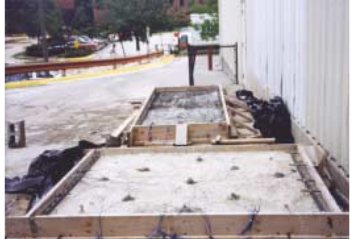
Fig. 4: Thermocouple layout before casting overlay
