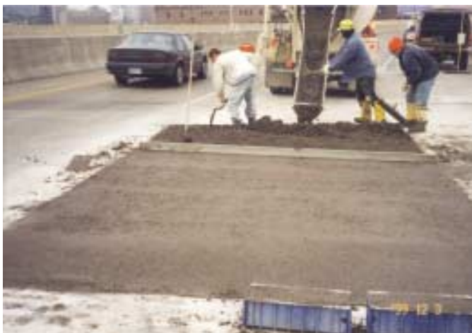
Fig. 1: Conductive concrete patch on an I-480 bridge deck
