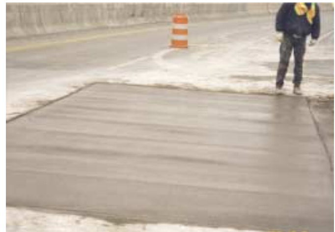
Fig. 2: The conductive concrete showed excellent workability and surface finishability
