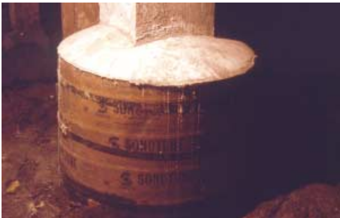
Fig. 7: Shear collar reinforces column-footing junction
