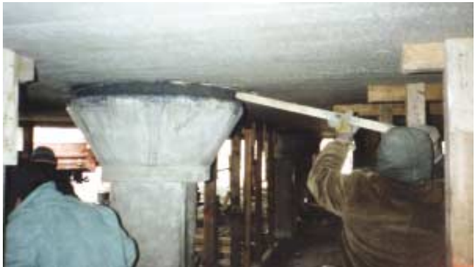
Fig. 2: Dry packing concrete between poured-in-place collar and slab soffit
