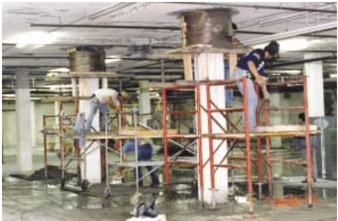
Fig. 4: Installation of shear collars using cardboard forms
