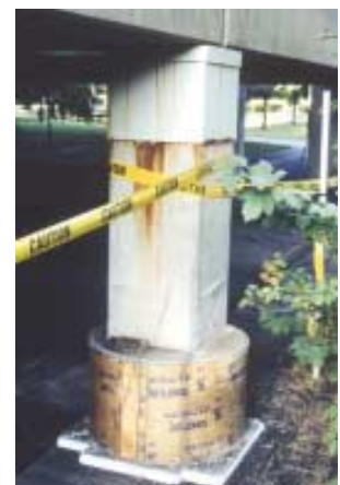
Fig. 11: A shear collar confines column reinforcing for seismic retrofit
