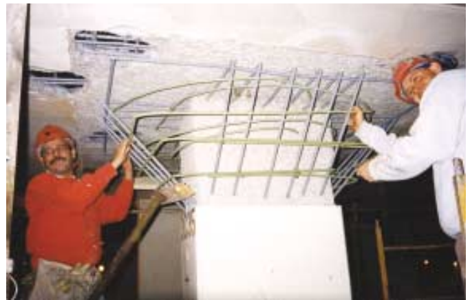
Fig. 6: Circular reinforcement is needed if a supplemental flaired column capital is to function as a shear collar
