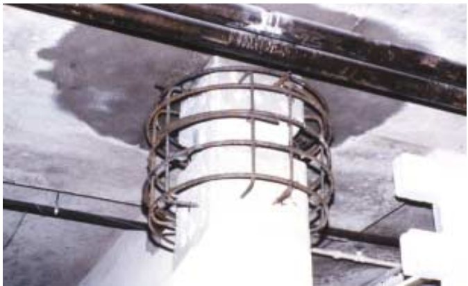
Fig. 3: Collar reinforcement in place before form placement
