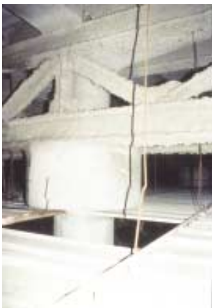
Fig. 9: Shear collar supporting a steel truss for supplemental floor framing
