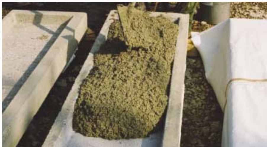
Fig. 2: Repair of simulated spalls in precast concrete slabs
