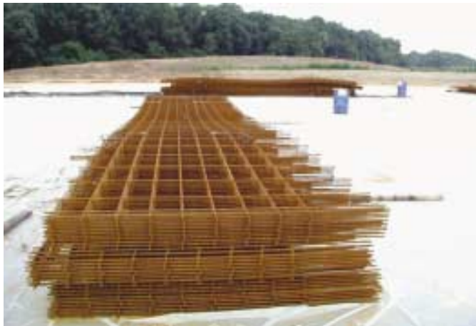
Fig. 1: Welded-wire reinforcement (WWR) bar mats (Photo courtesy of CON/STEEL Tilt-Up Systems, Dayton, Ohio)
